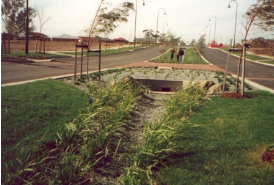
Landscape measures used in conjunction with infiltration in the centre of a boulevard
