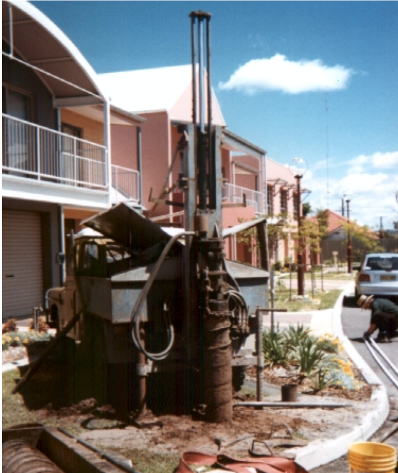
Installing a groundwater bore
